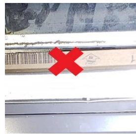
This filter is not.
